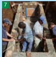
EKF1 Biogas Digester Project, Karagwe, Tanzania
